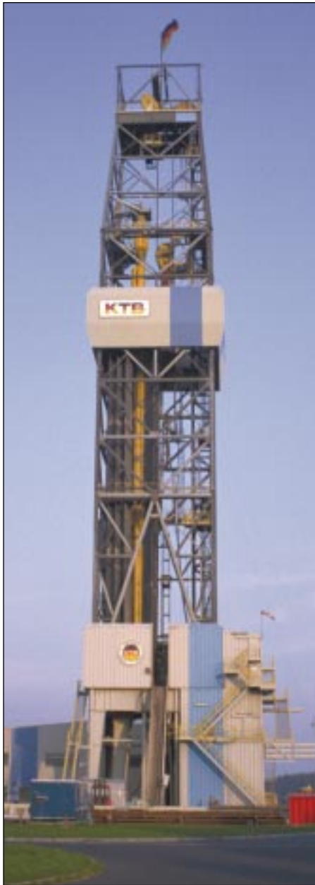
□ UTB 1. This is the largest land rig in the world, capable of drilling to 12,000 m [39,500 ft] and of handling extra-length drillpipe racked in stands of 40 m [130 ft]. The rig has many advanced features, including full electric drive, a large degree of automation and soundproofing.
